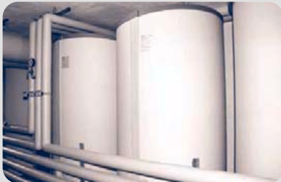
Solar thermal storage tanks
