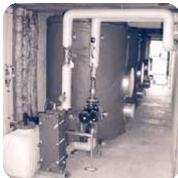
Boiler room with solar heat tanks, auxiliary heating and control unit
