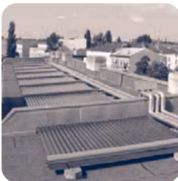
Horizontally mounted vacuum tube collectors on flat roof
