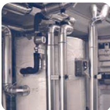
Vacuum-tube collectors and solar storage tank of the car centre Špan
