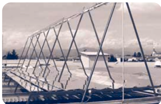
Fresnel collector for a solar cooling system in Bergamo, Italy Photo: PSE
