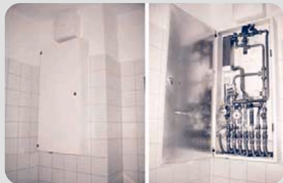
Fresh water unit in a building's two-pipe heating network. Apartment building in Salzburg.
