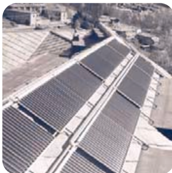
Vacuum-tube collectors on the roof of the retirement home in San Germano Chisone
