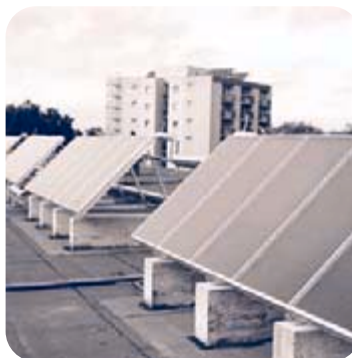
40° installation on flat roof
