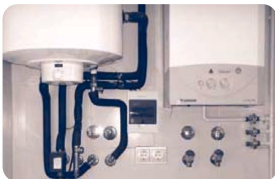
Solar heat storage, auxiliary heating unit and control unit in each flat in an apartment building in Spain.
