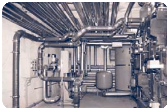
Centralised heat control station for solar and conventional heat
