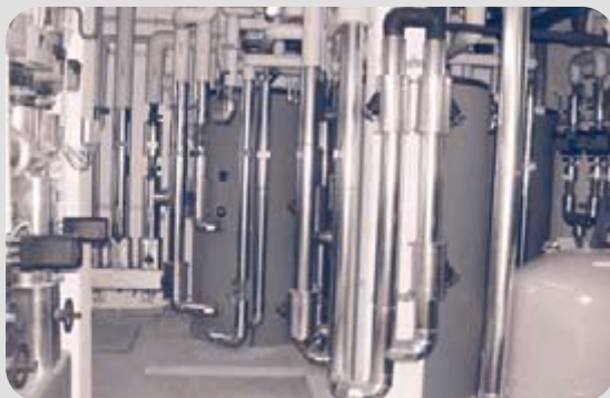
Boiler room with solar heat storage tanks and control unit
