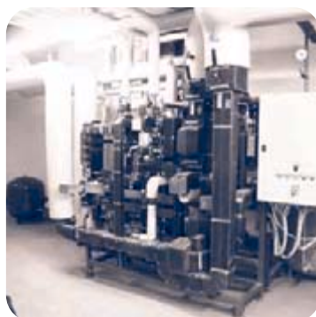
Combined solar energy and boiler control station "SEZ" in Berlin
