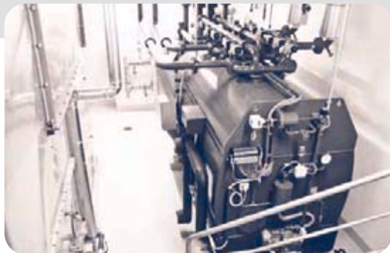
Solar air conditioning – adsorption chiller in the university hospital, Freiburg
